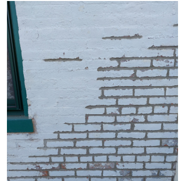
Recent tuckpointing work at the Farmhouse
